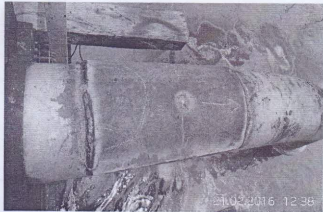
Figure 2: Repair on the Pipeline
